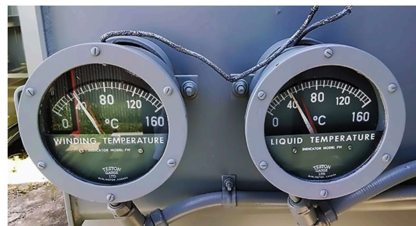
Oil and winding temperature gauge for overload protection
